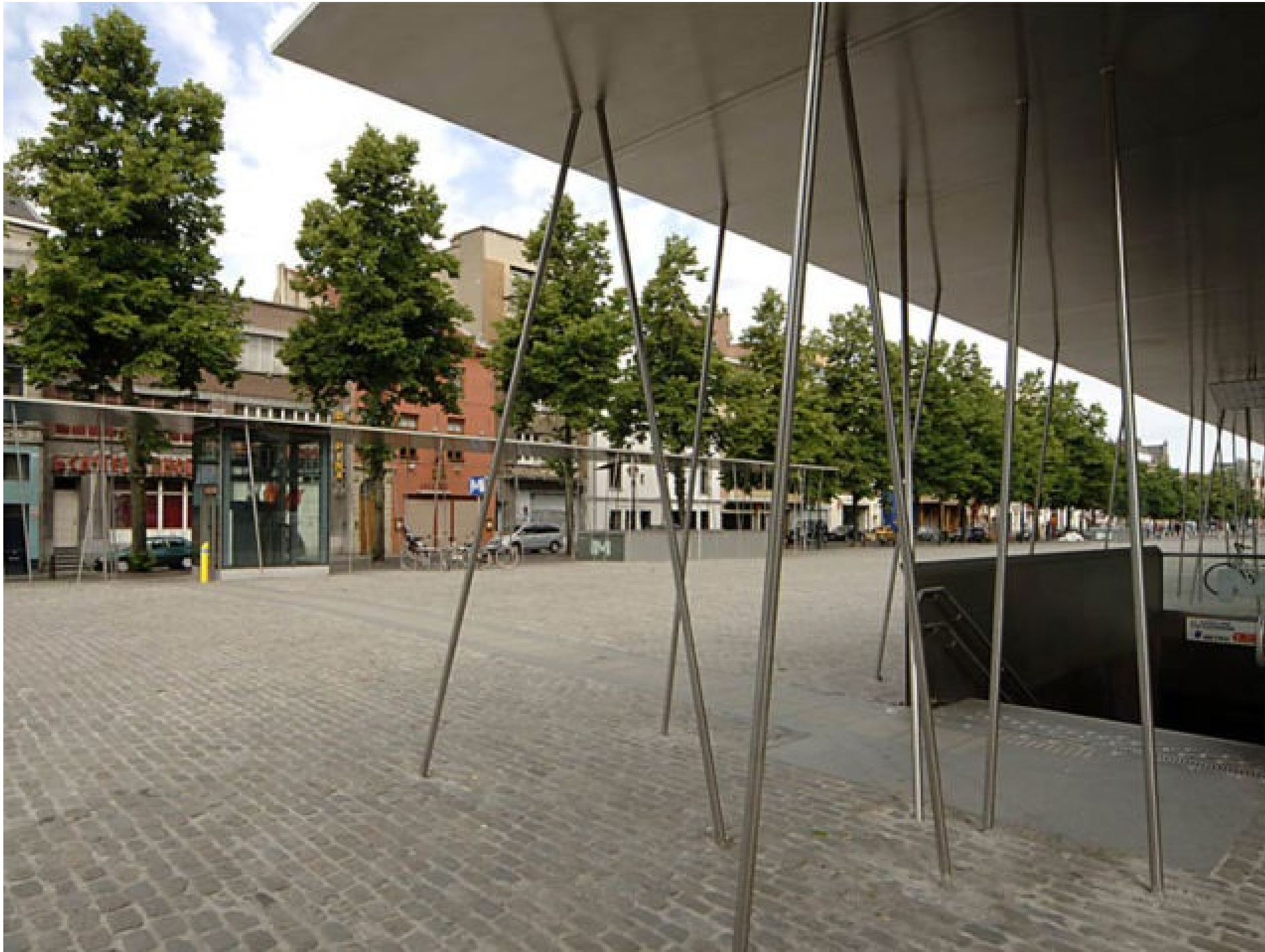
U-Bahnstation Sainte-Catherine, Brussels, 2007, Arch.: Olivier Noterman und Nicolas Vanden Eeckhoudt, Ing.: Ney and Partners
