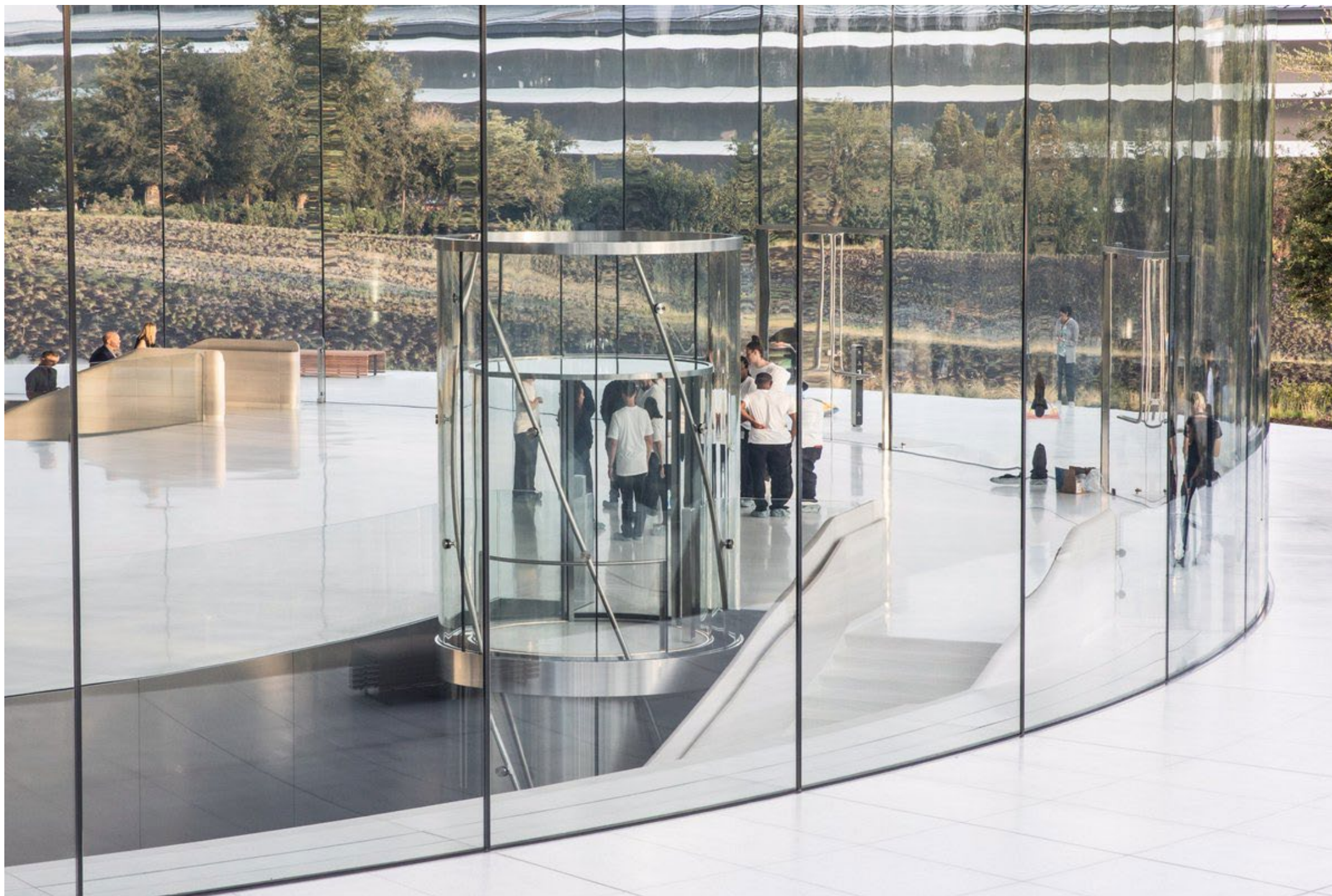
Steve Jobs Theater, Cupertino, 2017, Arch.: Foster + Partners, Ing.: Eckersley O'Callaghan
