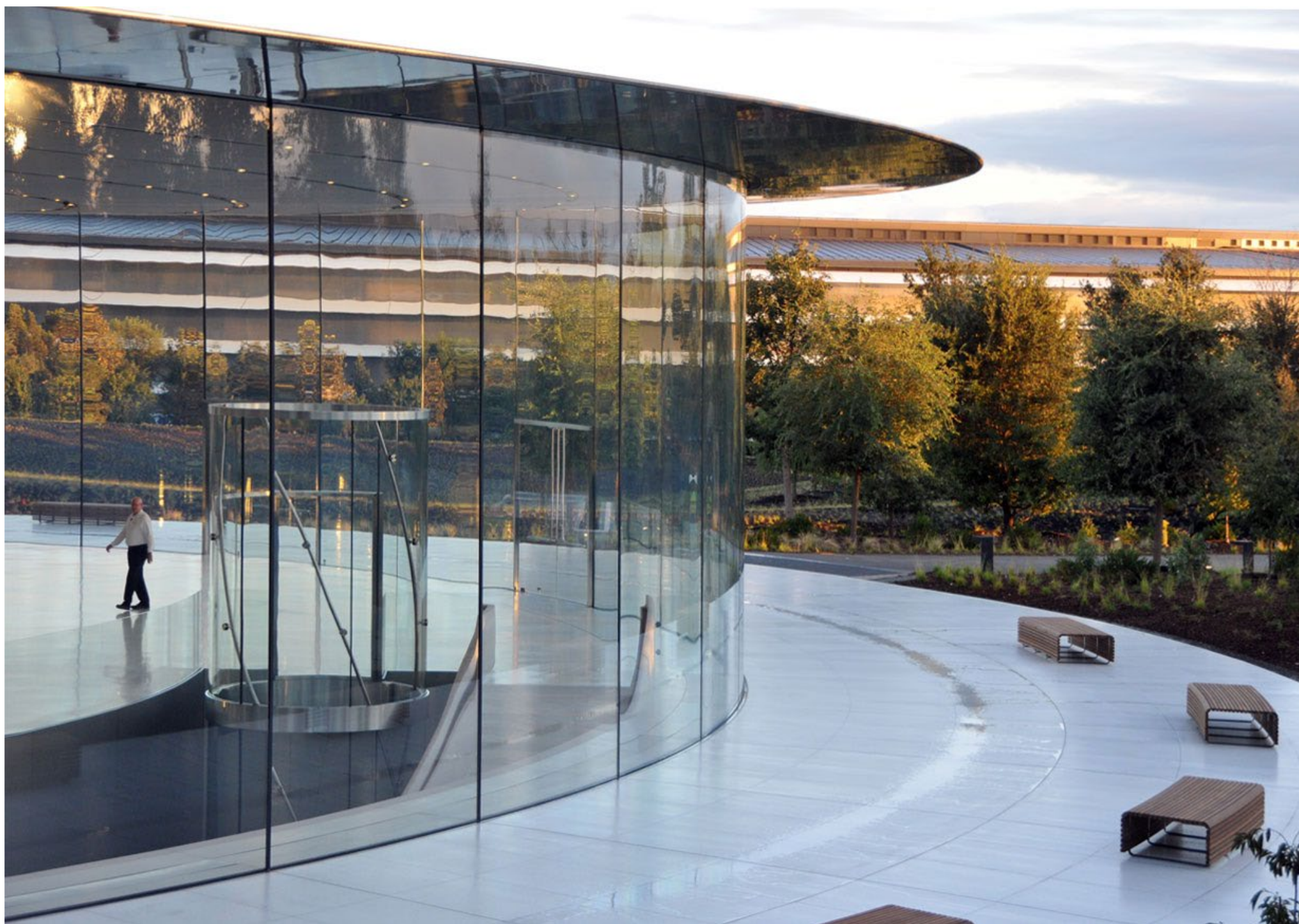
Steve Jobs Theater, Cupertino, 2017, Arch.: Foster + Partners, Ing.: Eckersley O'Callaghan
