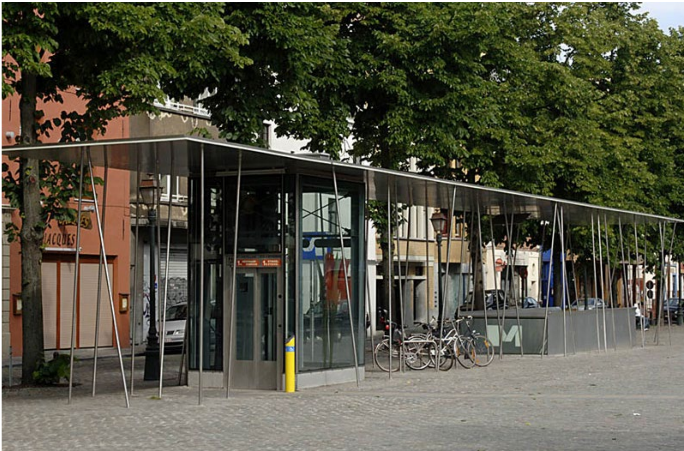
U-Bahnstation Sainte-Catherine, Brussels, 2007, Arch.: Olivier Noterman und Nicolas Vanden Eeckhoudt, Ing.: Ney and Partners
